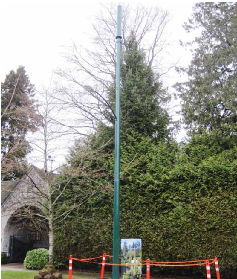
Example 1 of 13-metre tall streetlight antenna pole with connection cabinet at grade
