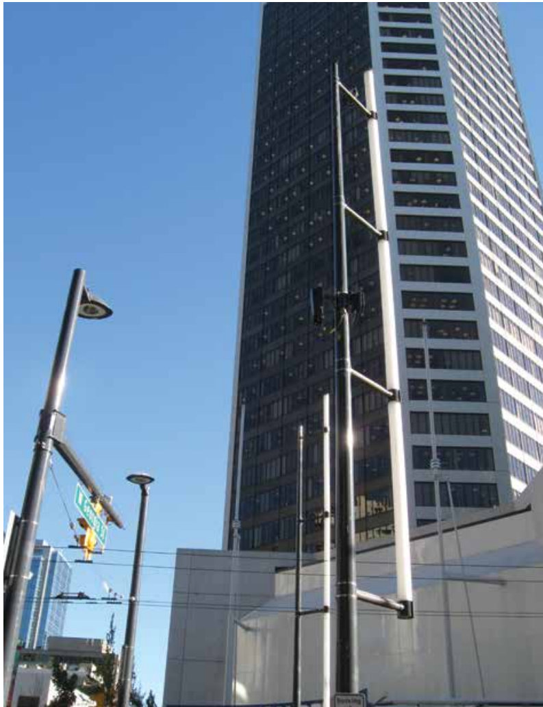
Small cell attachments to decorative street lights (the white vertical element is the light)
