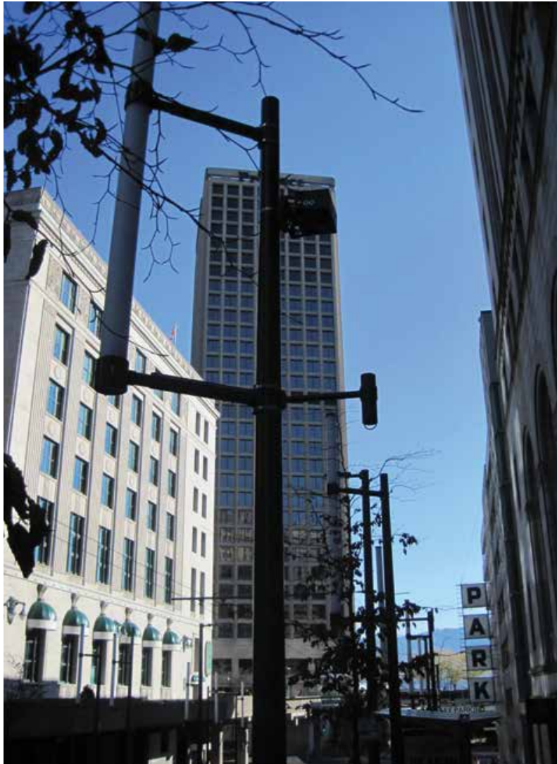
Small cell attachments to decorative street lights (the white vertical element is the light)
